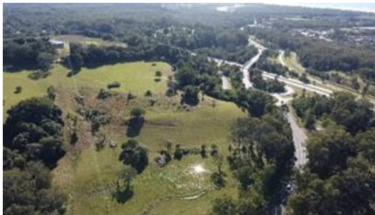
Area 5 looking over interchange.
